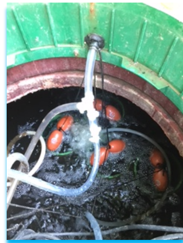
The ... RioVation® TRUE AEROBIC® ATU Conversion Kit Fixed Film Media (FFM) installed into an existing septic tank & operating.
